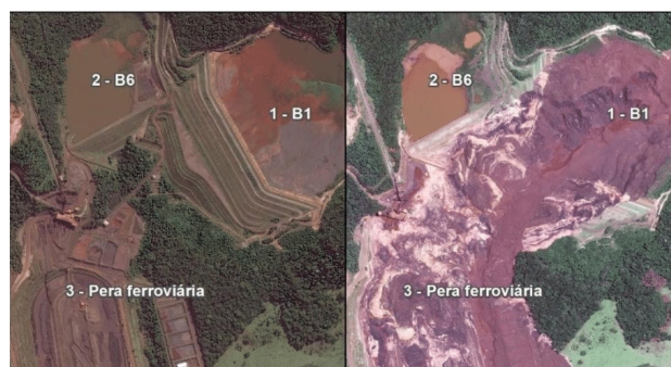
Figure 4 Detail of part of the affected area before and after the rupture.
